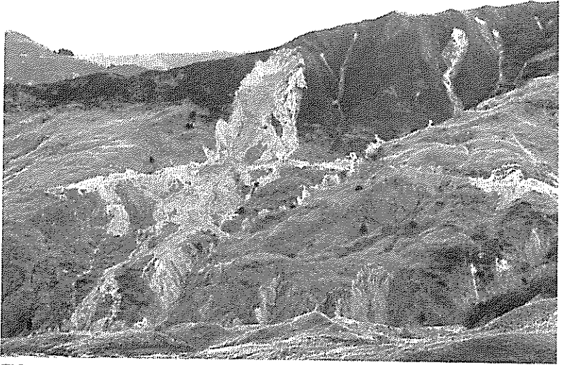
FIG. 4—Large debris avalanche which destroyed part of N.Z. Forest Service Road No.5, Owheua.
