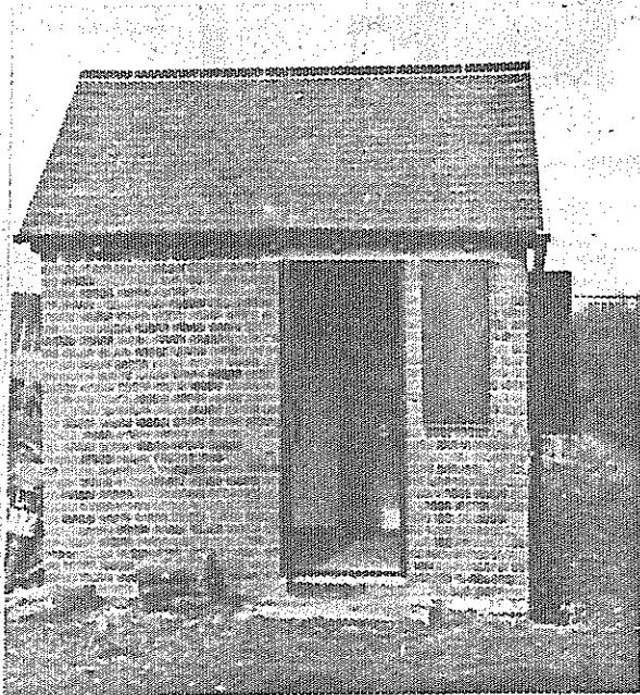
Fig.1. English cableway housing
