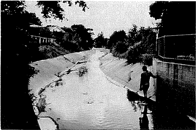
FIG 13—The enlarged and concrete-lined channel of the Wairau Creek immediately downstream of the Alma Road gauging site.
